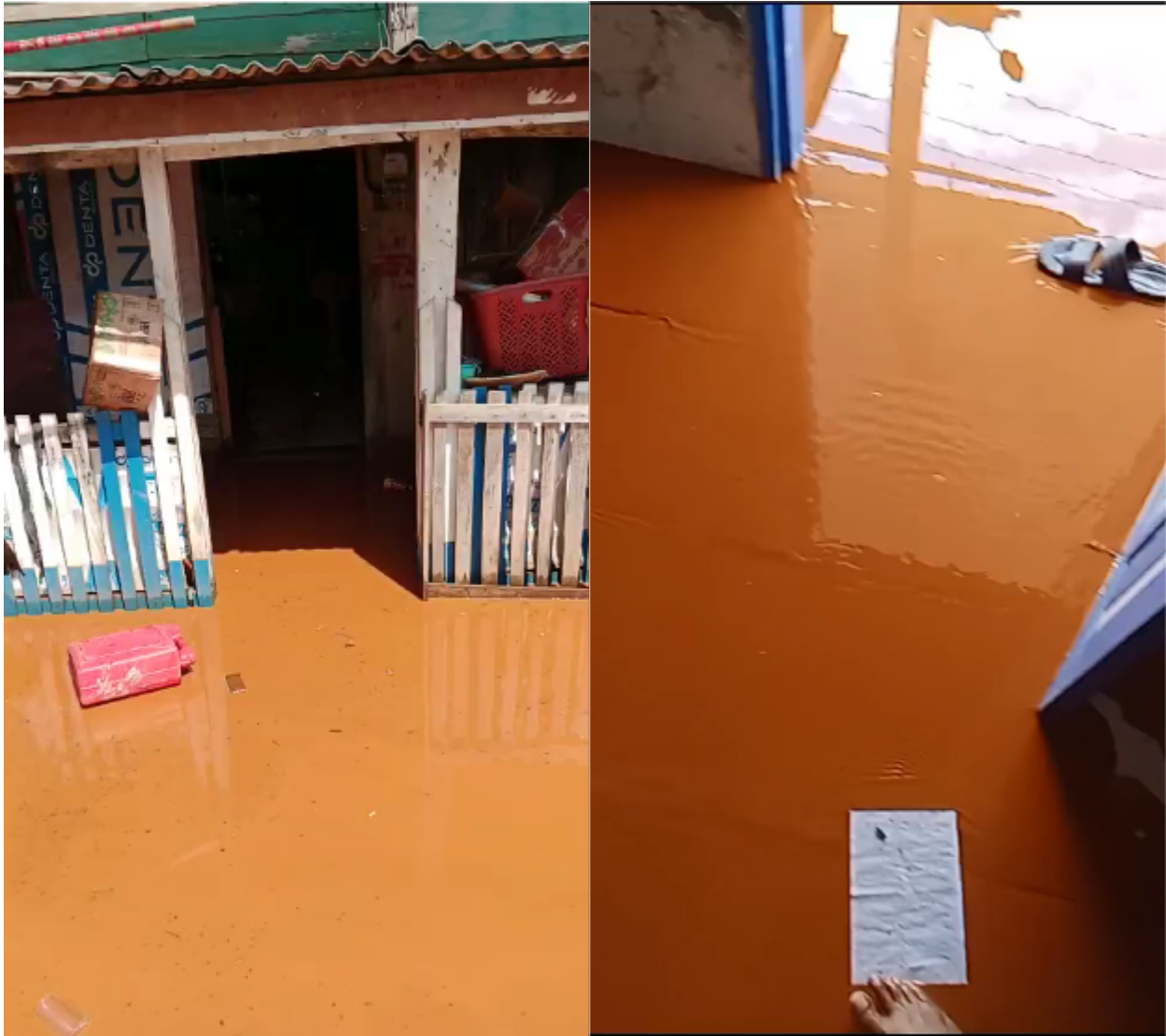
Photos: Flooding incident in Baliara area, West Kabaena, Southeast Sulawesi occurred after only half an hour of rainfall on Tuesday, 26 March 2024.
